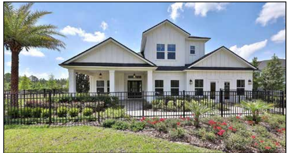
Photos provided by Beacon Lake
